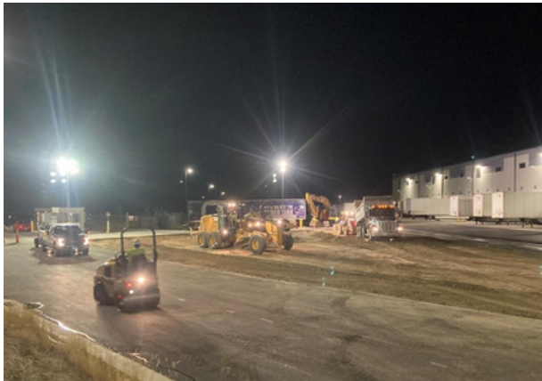
Contractor's Excellence Private Sector Under $10 Million Ontrac Pavement Repair
