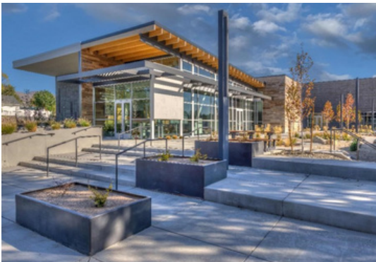
Contractor's Excellence Public Sector Under $10 Million Great Basin College Winnemucca Health Science and Technology Building
